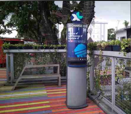
Charging Tower - Teras Cihampelas
